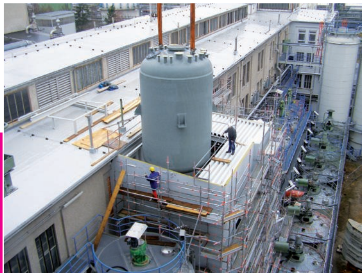
New polymerisation vessel for producing paste PVC in the expanded paste plant in Burghausen
